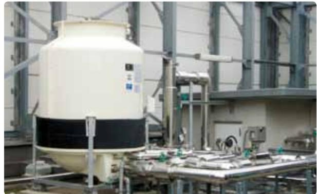
As calcium and other solids do not evaporate, they remain in the cooling tower circuit. When make-up water is introduced, the solids remaining after its evaporation add to the already existing solids - building up more and more. Problems then occur, as these built-up solids typically clog up the system.
